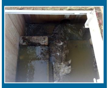
Figure 1: CSO spilling litter due to blocked screen
