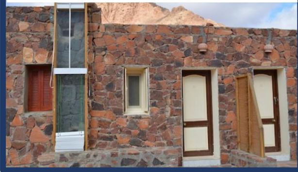
Figure 2 The Trombe wall ventilation system (left) has been modified to be used both for heating and cooling using renewable energy sources. Researched by Marwa Dabaieh from Lund University in Sweden. Tested in Saint Catherine, Egypt Photo: Insaf Ben Othman
